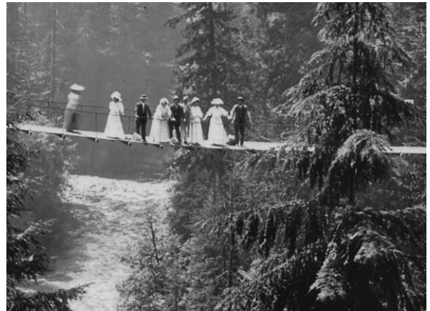
Named for the Squamish word which means “beautiful river,” the first version of the suspension bridge was erected in 1880. The gorge is an exhilarating wonder of natural beauty. Even with all the modern steel cabling,
