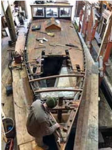
Stripping the old deck. Photo courtesy of T Burnett.
