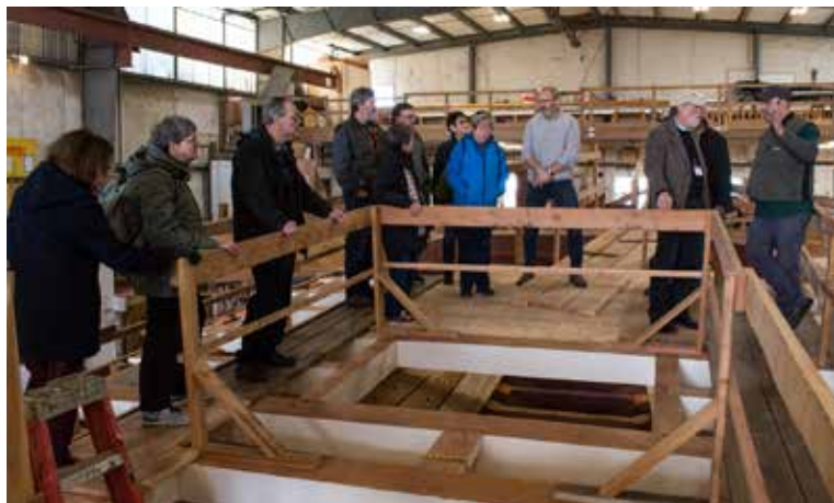
Looking down into the hull of the Western Flyer as Chris Chase (grey shirt), Project Manager for Western Flyer Foundation, and Tim Lee (green hat), Partner, Port Townsend Shipwright's Co-op and Lead Shipwright responsible for the renovations, lead a small group. photo: ET Becker
