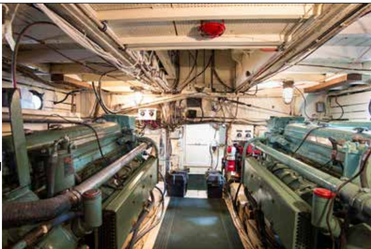
Inspecting the engine room on Annie Laurie . photo by M Fazio
