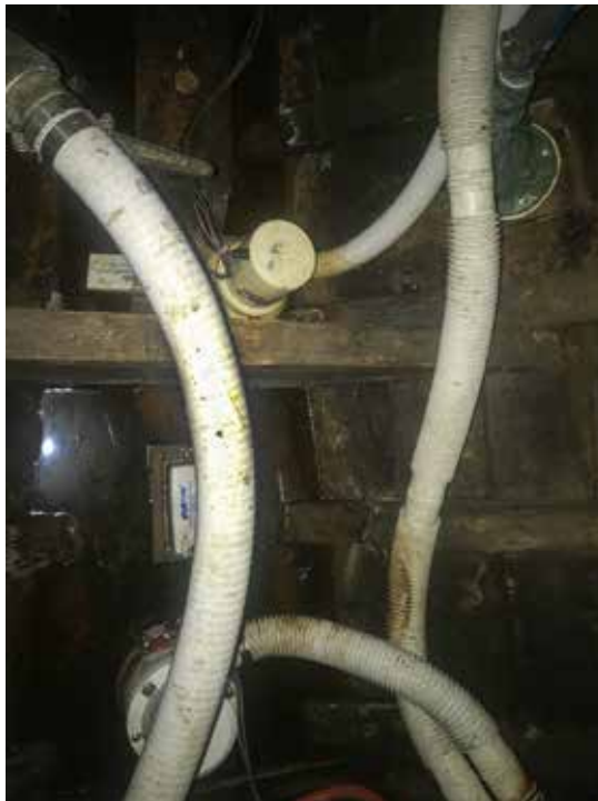
Inspecting the forward bilge pumps through the hatch on Annie Laurie . photo by M Fazio
