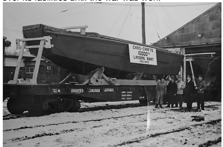
Emblematic of Chris-Craft’s immense contribution to the war effort during World War II is this photo of its 10,000th landing craft leaving the factory in early 1945. photo from Chris-Craft archive.
