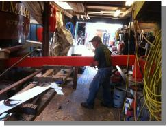
The new timber was coaxed in over the deadwood and new bolt tops were driven down the pre-bored holes and welded to the old bolt stubs from the protruding deadwood. The new horn timber was then dogged down onto the deadwood and a new transom knee was fitted over the old bolts in the transom, keeping undisturbed.
