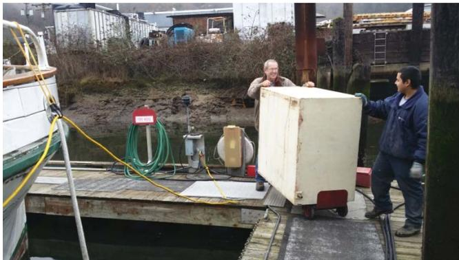
Old steel fuel tanks being removed. Water tanks removed to be cleaned and reused.
