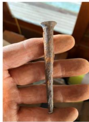
What remains of an 88 year old ferrous bolt. The remaining 1/4” of the bolt was still doing its job and strenuously resisted being removed.
