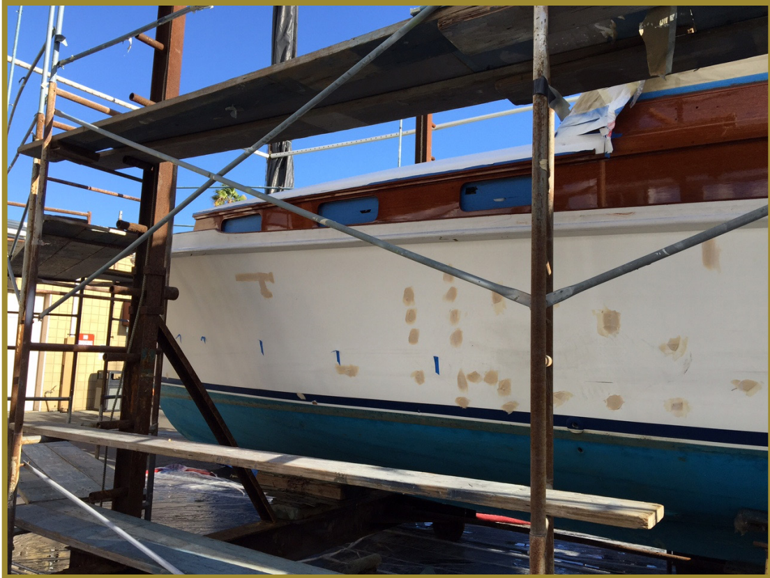
Minor repairs around the waterline, aft and deck areas were done using West epoxy systems.
