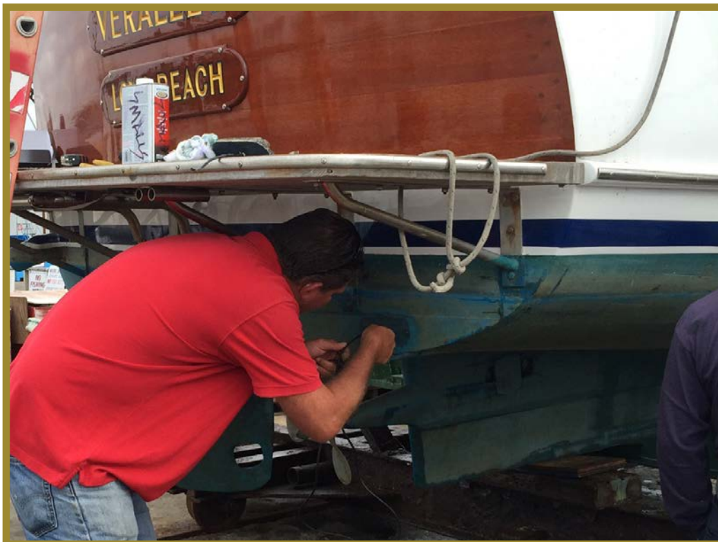
Repairing the underwater lights
